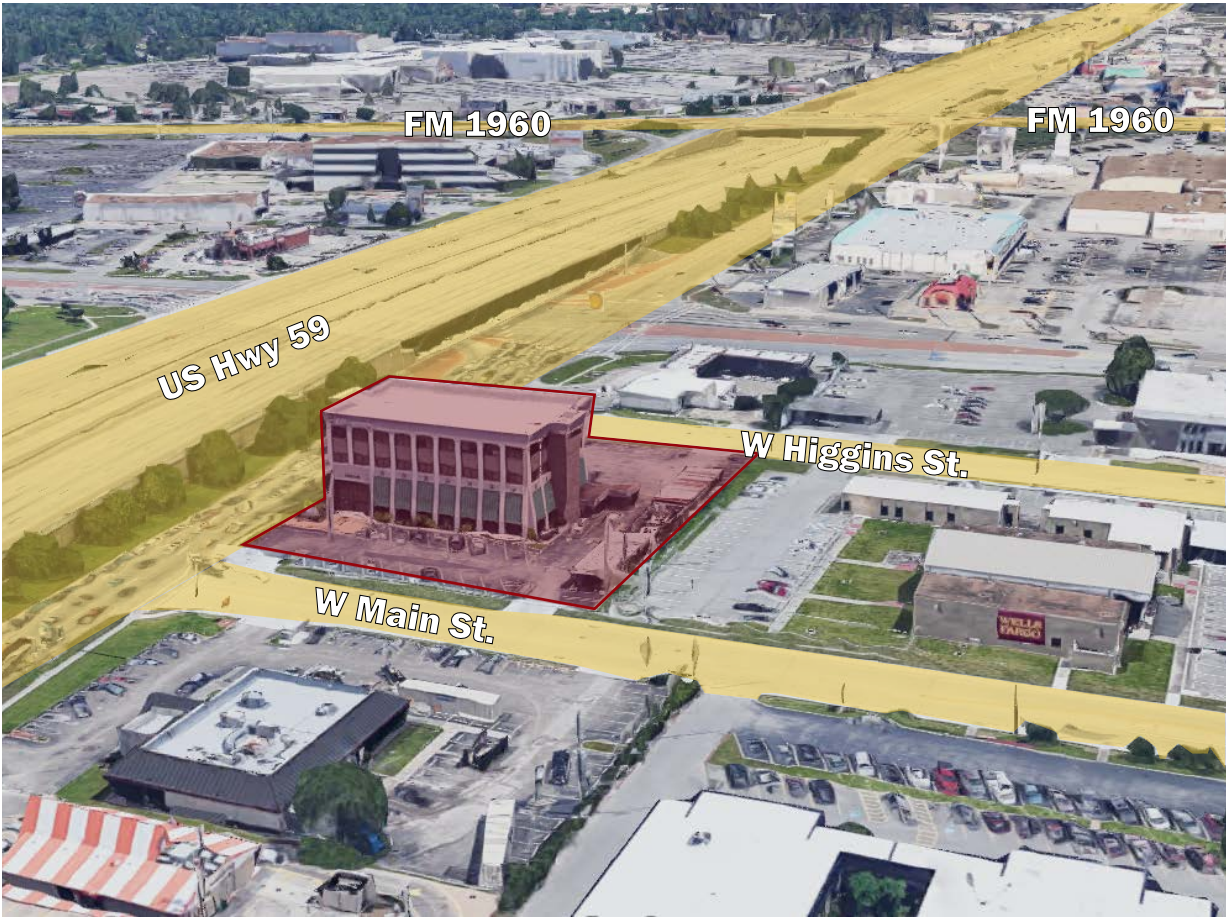
Office space for lease in the three-story Plus4 Credit Union building in downtown Humble. Vacant space available on the first, second and third floor.
